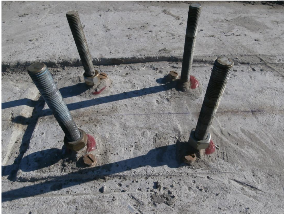
Figure 22: Epoxy Anchor Replacement for Anchors Installed in Rotated Positions
