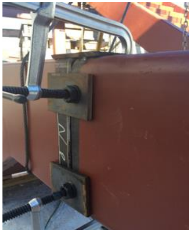
Figure 16: Splicing HSS of Unequal Wall Thickness
