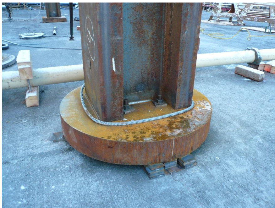
Figure 18: Narrow Anchor Rod Pattern Causing Erection Stability Issues
