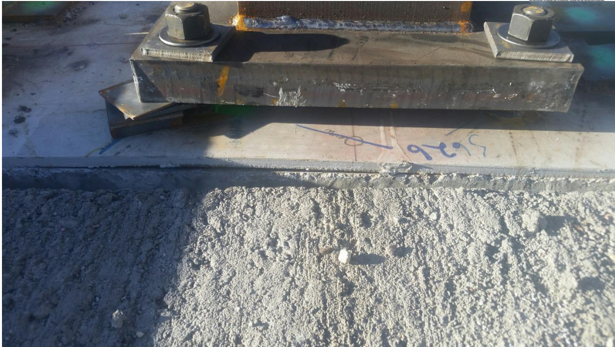
Figure 21: Embed Plate Failure from Wind on Anchor Rod Tensile Loads
