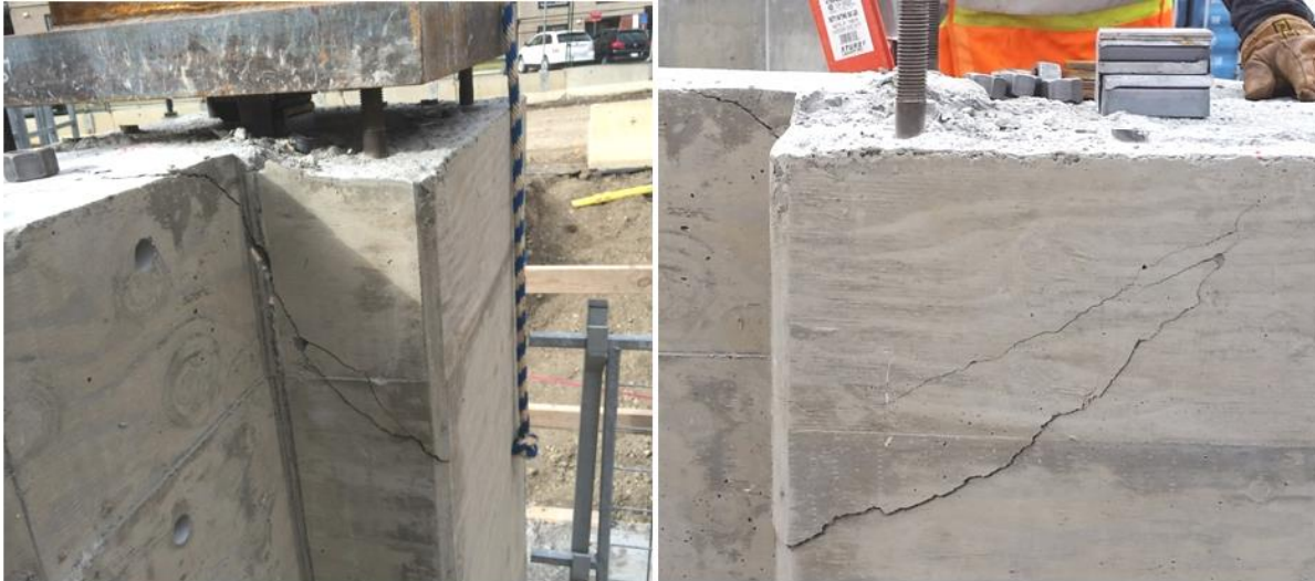
Figure 19: Base Plate of Similar Size to Concrete Pier with Anchor Rod Failure
